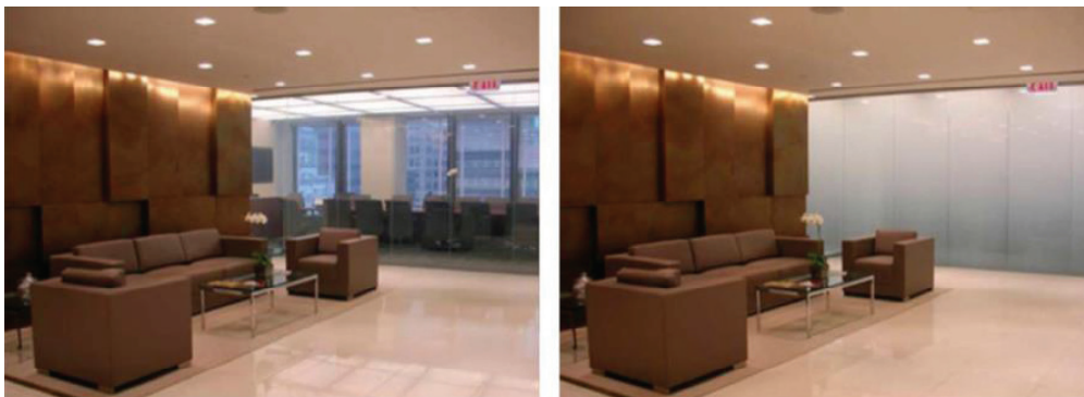
Fig. 12. PDLC operating modes: transparent mode and dark mode, respectively (Source: Rezaei, 2017)
